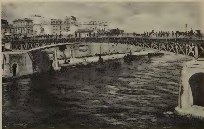
The iron swing bridge across the canal at Taranto, Italy, which admits the largest war-vessels. The seaport was an important naval base in the war.
